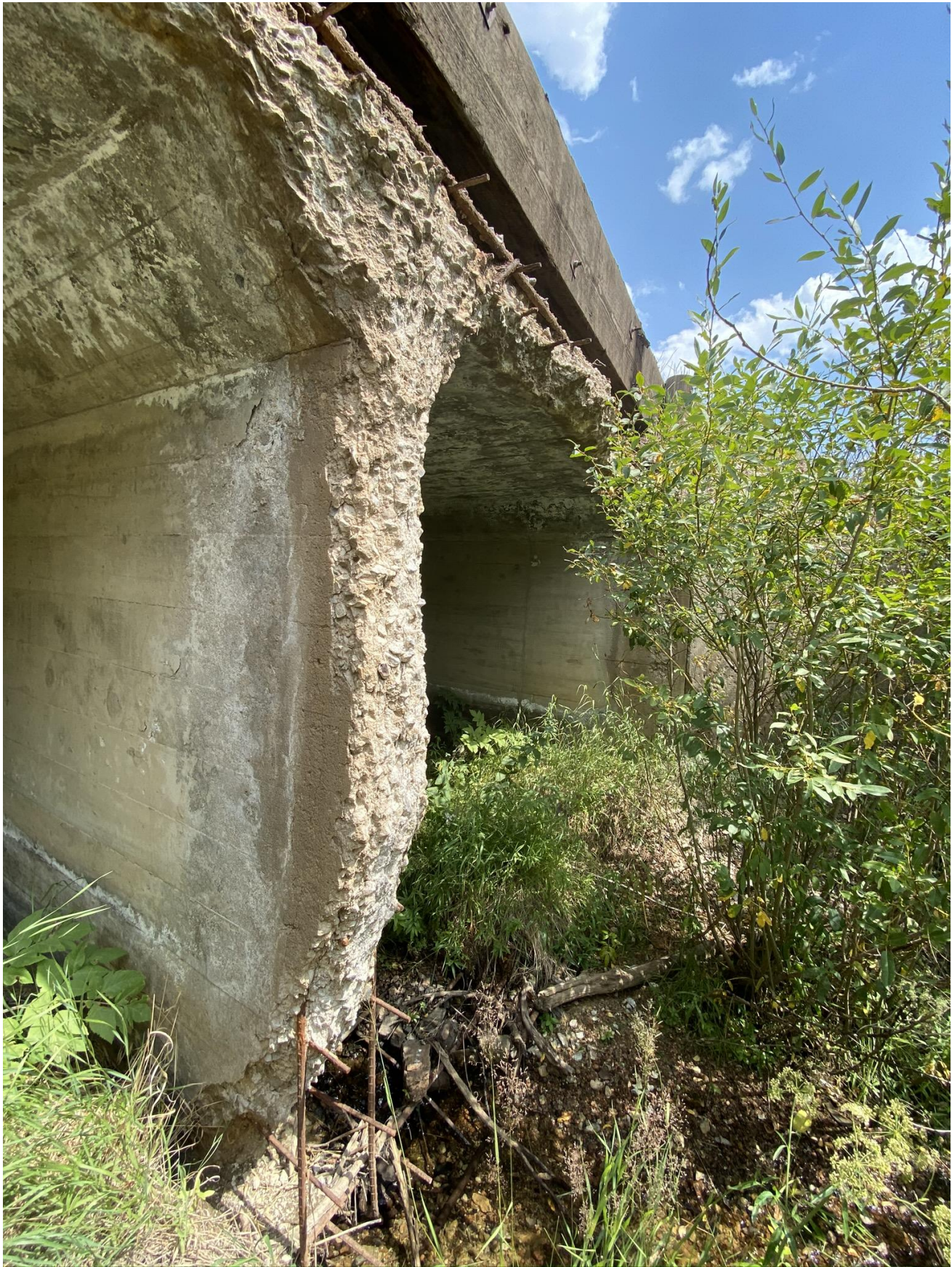
EXISTING RCBC STRUCTURE STREAM ABRASION STRUCTURE I-15-T FIGURE 1
